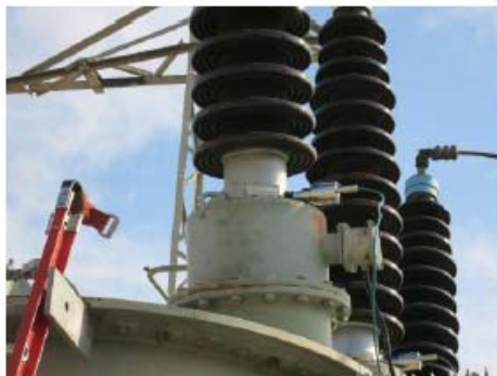
Fig. 11 Bushing adapters for on-line PD measurement
